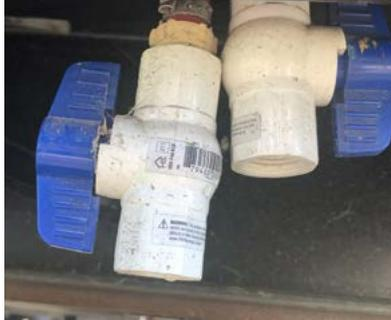
Next, run the water pump for a bit to help force any water out. Turn the water pump off as soon as the water has drained. Be careful not to run the water pump without any water in the system for too long, or you might ruin the pump.
